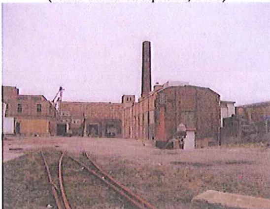
West Elevation (Photo Taken on April 27, 2007)
