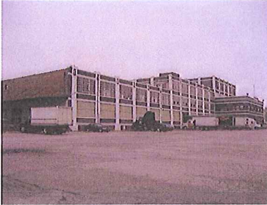
Southeast Elevation (Photo Taken on April 27, 2007)
