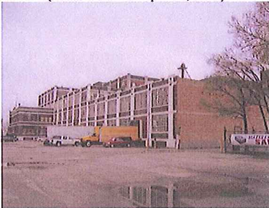
Northeast Elevation (Photo Taken on April 27, 2007)
