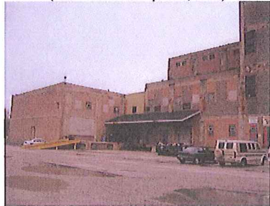
North Elevation (Photo Taken on April 27, 2007)
