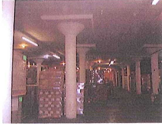
First Floor Warehouse Space (Photo Taken on April 27, 2007)
